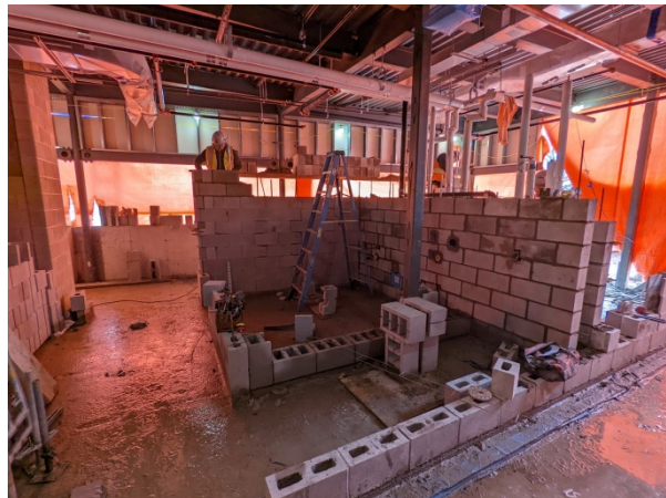
Interior: View towards the southeast (accessible change room)
